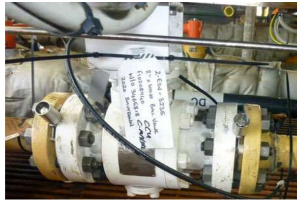
Alba-RIG™ test on ESVs – North Sea 2020
